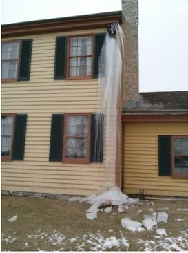
For the second winter in a row, the Colonel Davenport House has experienced large ice dams when thick ridges of solid ice build up along the eaves. Because of faulty routing of the furnace/air conditioning condensate removal piping, the water from the system cannot be dumped directly outside. We have a plan that will allow the routing of the condensate piping directly into the house drain without going outside.
