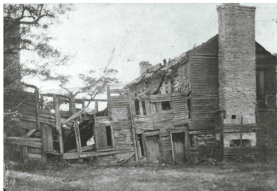
Kitchen Wing (looking west)
