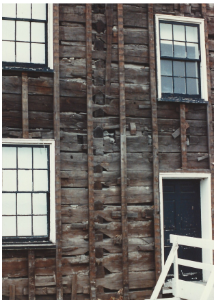
View of the log construction under the siding
